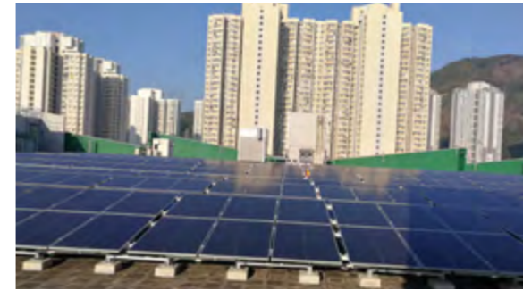
CREP puts into use the roof photovoltaic green energy utilization project.
